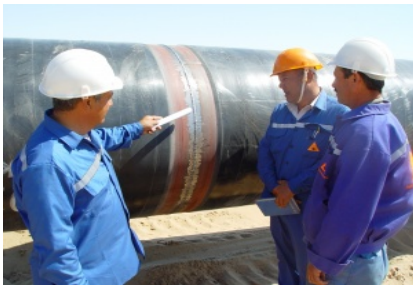
Turkmen Iran Gas Pipeline
